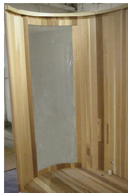
When in place, the first and second wall panels will look like this.
